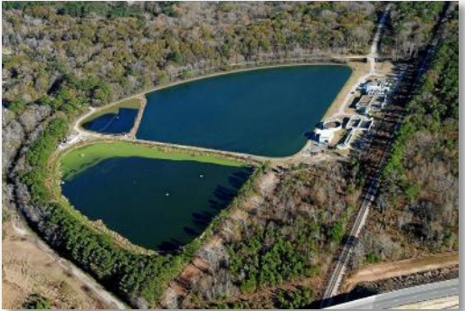
City of Pooler WWTP Membrane Bioreactor Upgrades
