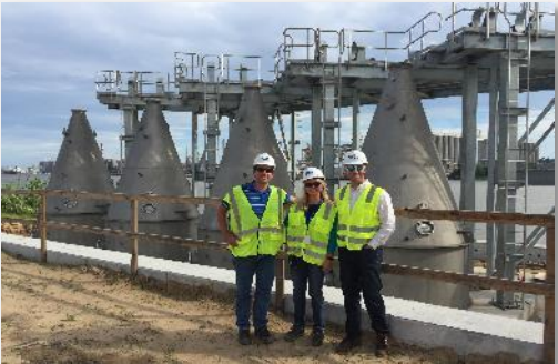
Savannah River Dissolved Oxygen Facility
