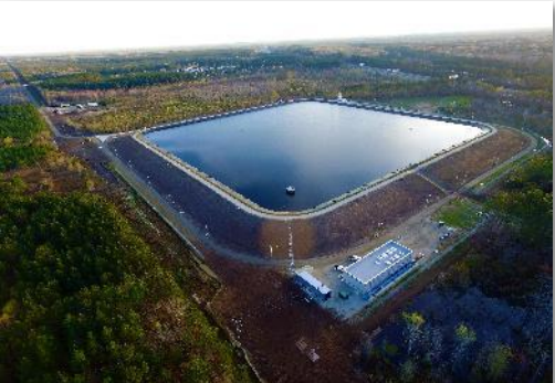
Savannah Raw Water Storage Impoundment
