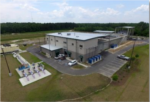
City of Richmond Hill Sterling Creek WRF
