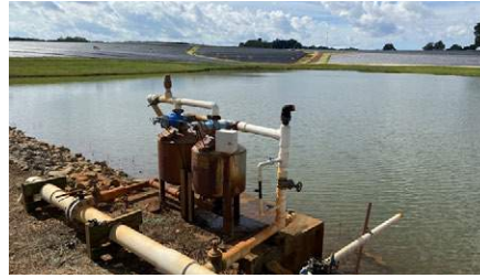
Spartanburg Water Advanced Oxidation Treatment System
