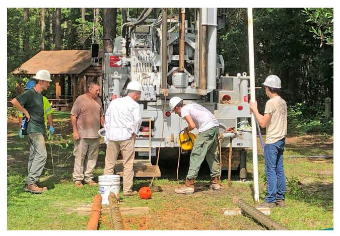
Figure 30. The South Carolina Geological Survey assisted in drilling a water-table well (COL-0803) at Colleton State Park in Colleton County.
