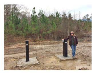
Figure 26. Two new monitoring wells at 8 Oaks Park in Georgetown County. GEO-0390 (right) is a 4-inch well, 640 feet deep and screened in the Crouch Branch aquifer. GEO-0391 (left) is one of the 10 monitoring wells drilled in late 2018 and early 2019 to monitor the surficial aquifer system throughout the Coastal Plain.
