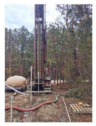
Figure 22. Installation of the 2" PVC well casings at the Sumter cluster site.
